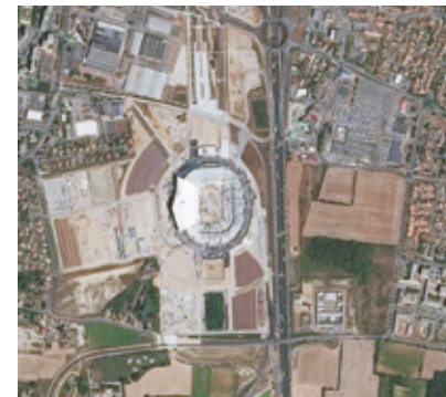
Construction of Lyon's new football stadium.
